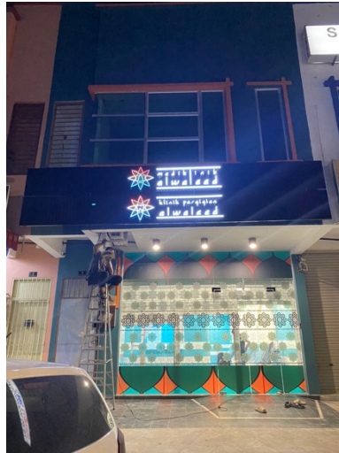
Figure 7. The image of the clinic entrance during construction
